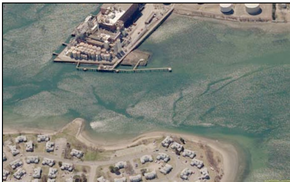
View of Twin Rivers Technology from the North
