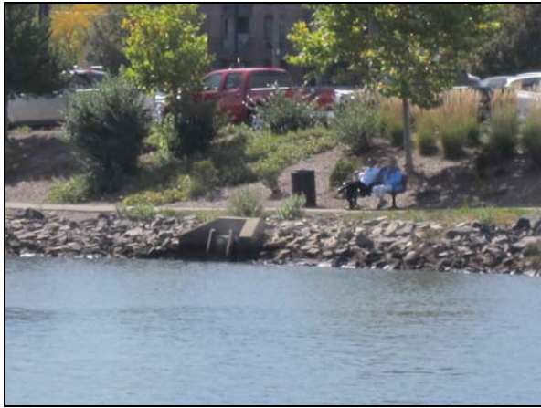
Culvert located near National Grid
