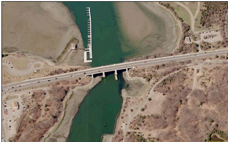
Looking North to the 3A Bridge
