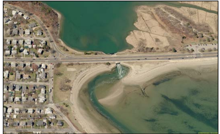
Tide Gate at Blacks Creek
