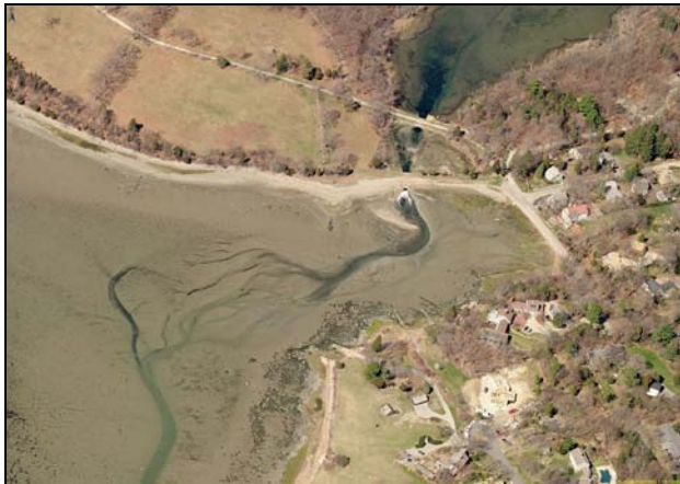
Culvert at CB02c
