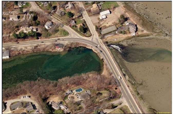
Culvert at CB02a
