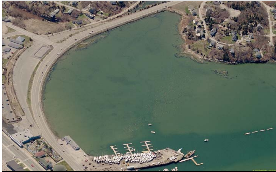
George Washington Blvd, both culverts are located in this area.
