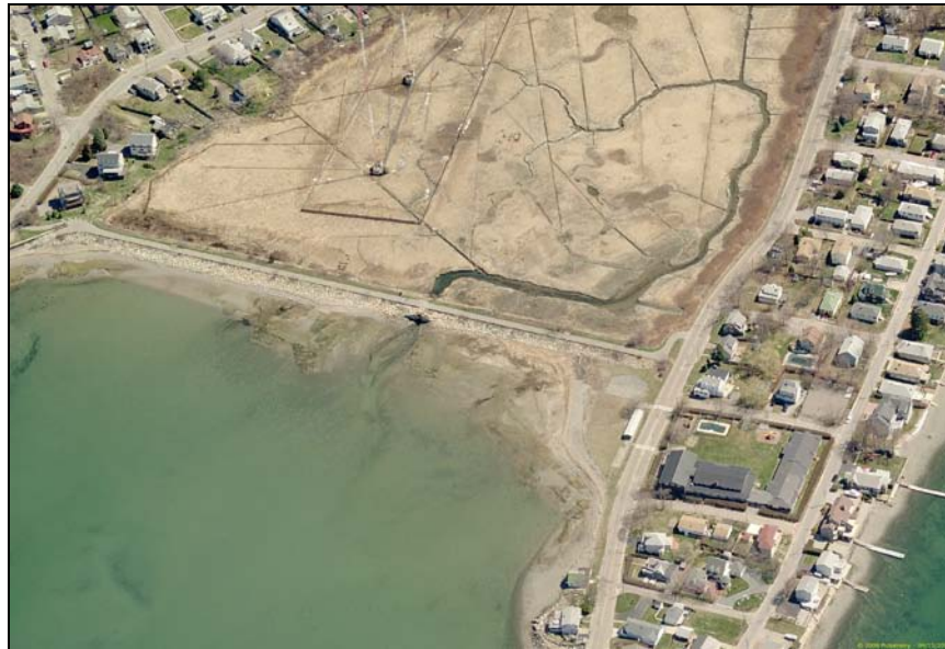
Tide Gate located along Nantasket Road.
