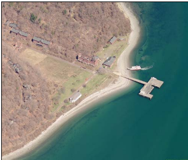
Dock located at the Northeastern point of Peddocks Island.
