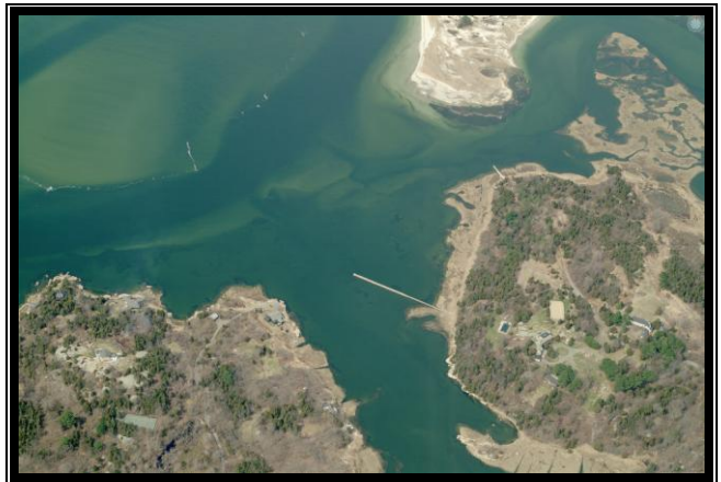
Entrance to Farm Creek. MassDEP, 09 April 2009.
