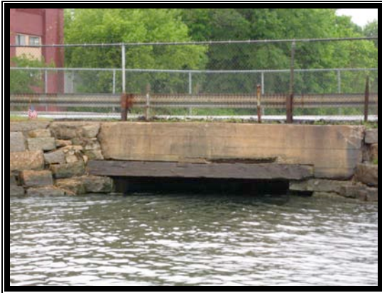
Liberty St culverts at high tide on 27 May 2009. View looks west.
