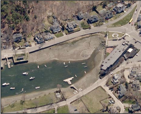
View looking southwest towards the tide gate near Elm Street. (TG)
