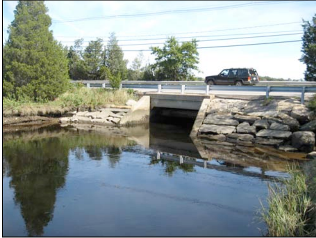
Culvert located along Gannett Rd.
