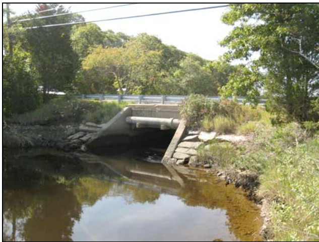
Culvert located along Gannett Rd.
