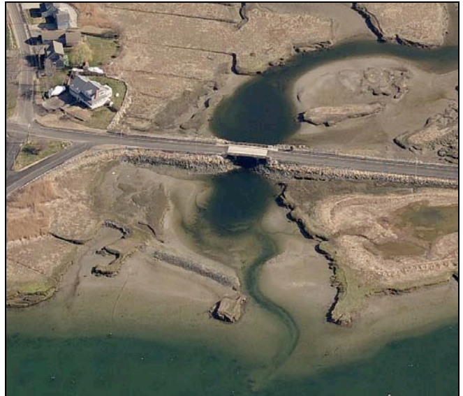
View looking south towards DV-01b.
