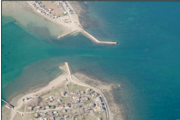
View looking north towards Old Scituate Lighthouse and shoreside recovery location.
