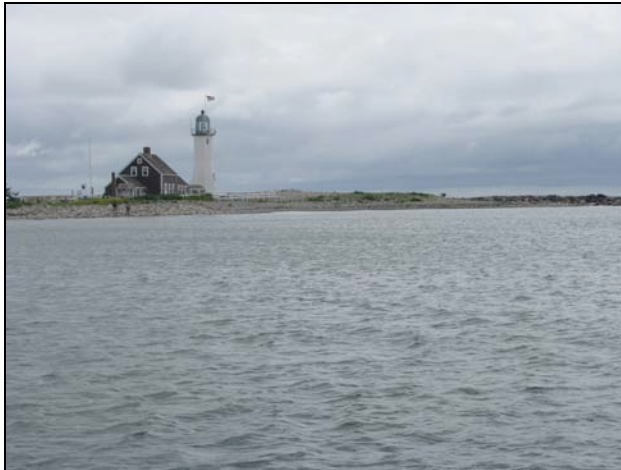
Shoreside Recovery area near the jetty by Old Scituate Lighthouse.
