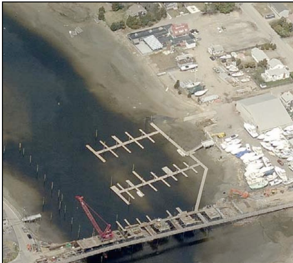
Boat Ramp located in SS-06 at Webster Street.
