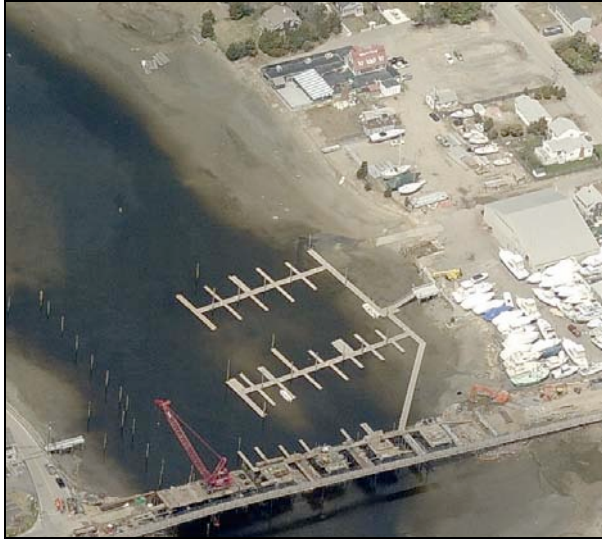
View looking north towards DV-01a and the boat ramp.
