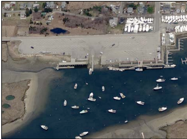
Boat ramp located on Town Pier Road.
