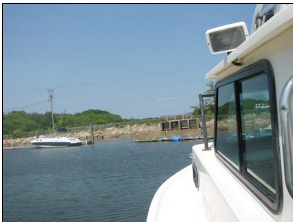
Tide gate located on Dyke Road.
