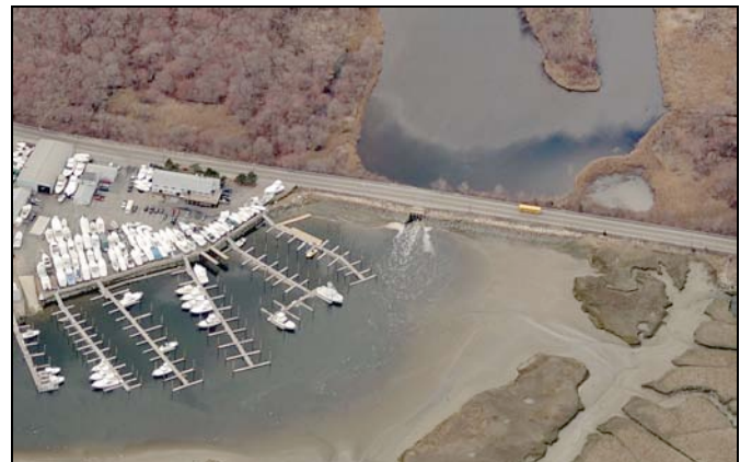
View looking west towards tide gate on Dyke Road.
