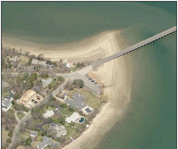
View looking northeast towards the boat ramp on Powder Point and the shoreside collection area for DV-01
