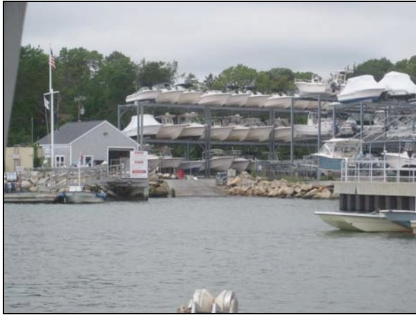
Boat Ramp at Bayside Marine Corp.
