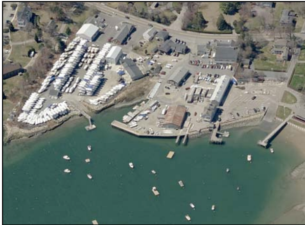
Looking West towards the boat ramps off Washington Street. (EX-02)
