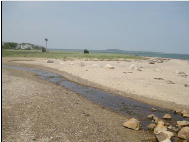
View looking north across the small creek at Nelson Park where the beach berming tactic would be constructed. (BB-02)
