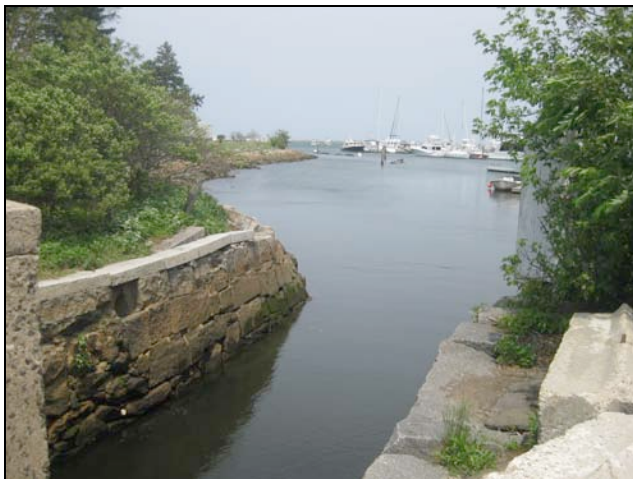
Culvert at Water Street.
