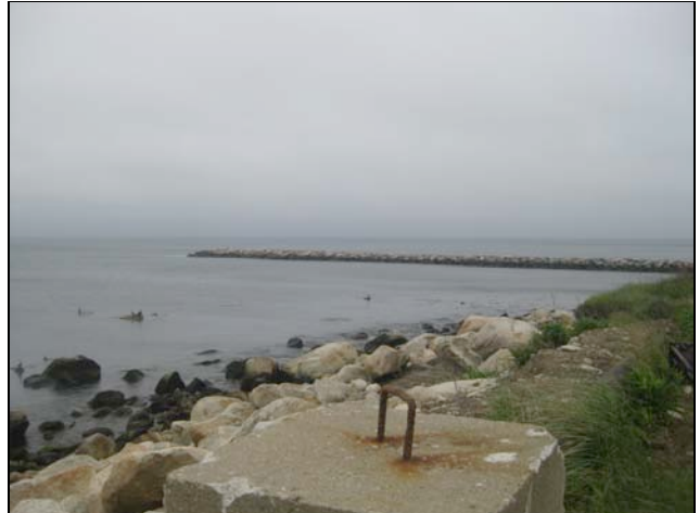
View looking south from the shore of the Pilgrim Nuclear Power Station intake lagoon. (EX-01)
