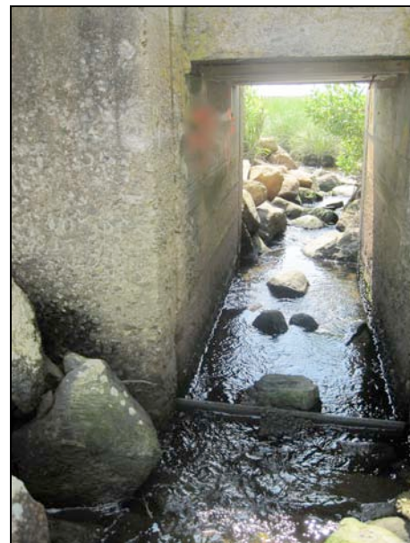
Culvert located near Ellisville Road. (CB-02)
